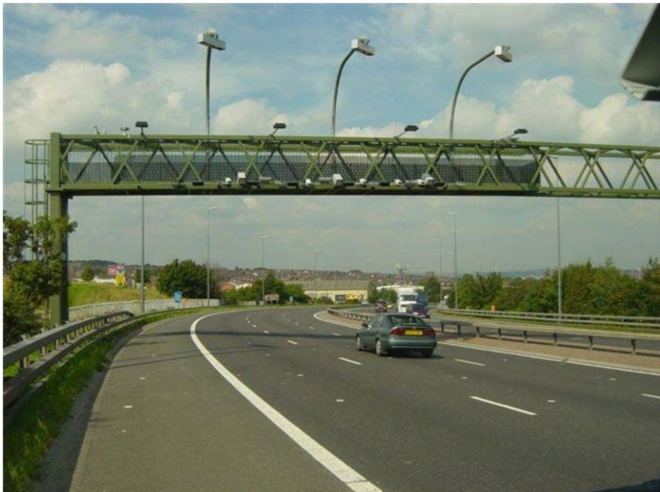
Figure 1 - Kapsch / Combitech solution to Road User Charging enforcement during on-road trials in Leeds (photo TRL)
